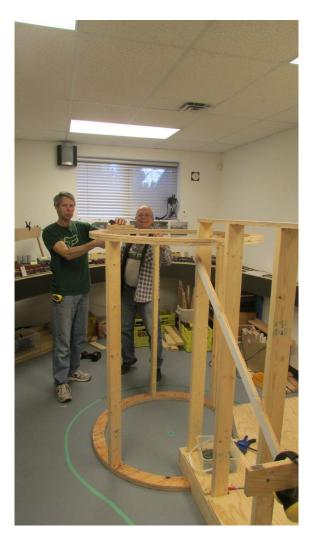
Detail showing the ¾ ring interfacing with the raised floor. The green ring shows the outside of the completed benchwork on the right the Chief Engineer is happy that the design has worked!!
