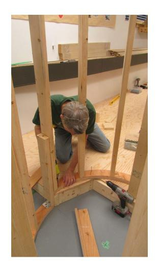
Once the cage is secured to the raised floor, the next task is to align and secure the new wall so it is straight and level.
